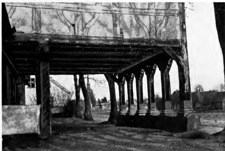
FARM-HOUSES IN LOWER VISTULA VALLEY SHOWING CHARACTERISTIC PORCHES, RELICS OF DUTCH AND LOW GERMAN CIVILISATION
